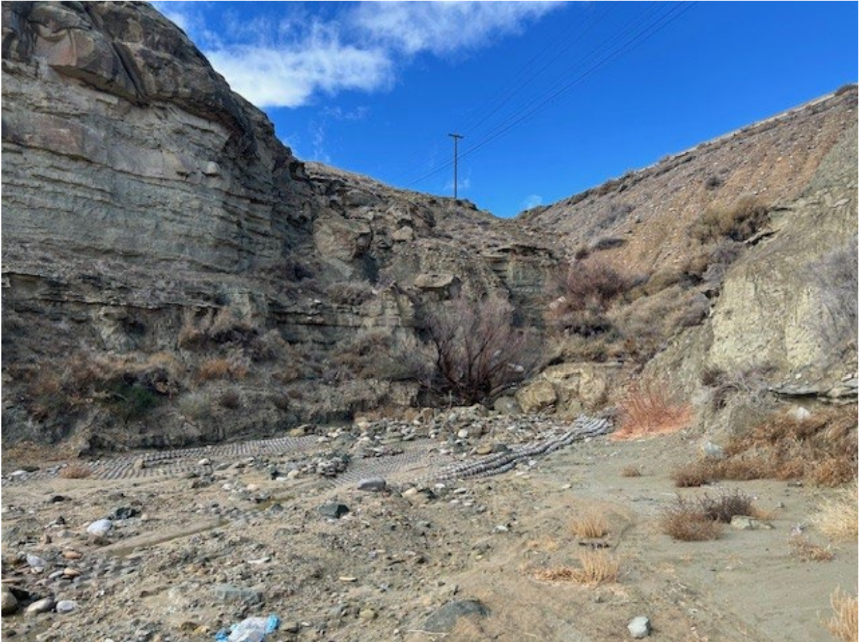
Figure 4. Damage to the ACB Matting
